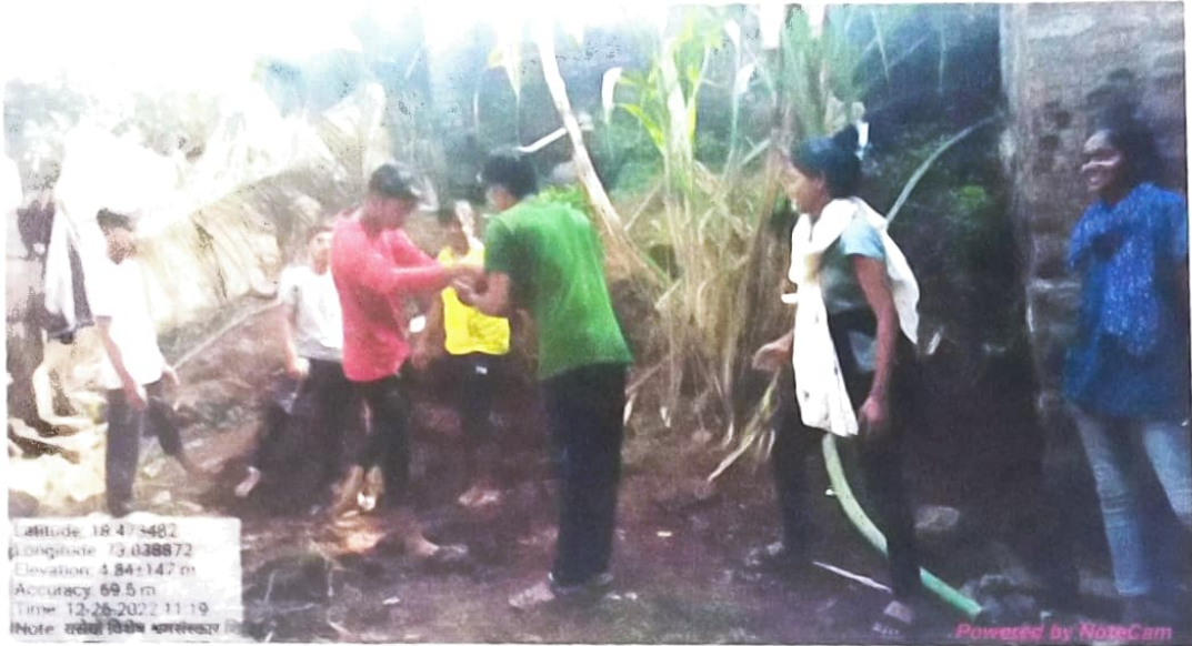
5. Students working for soak pit.
